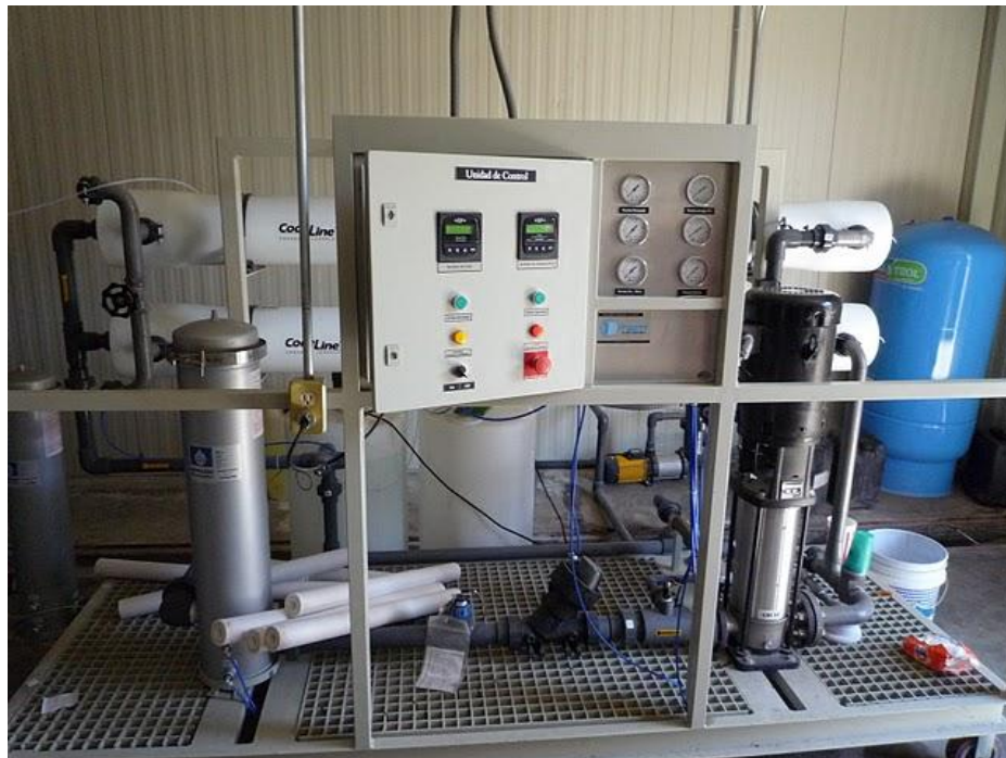
Water treatment plant in La Siberia, Zaragoza in the State of Nuevo Leon
