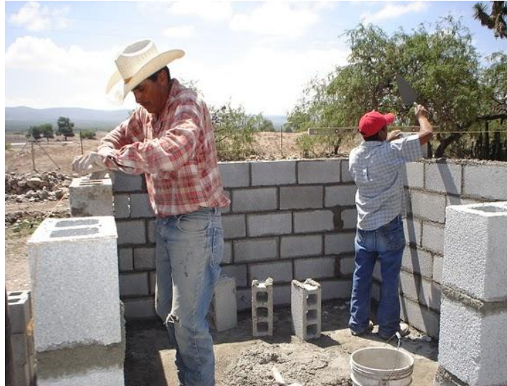
Local masons building wall to house the BYOW System
