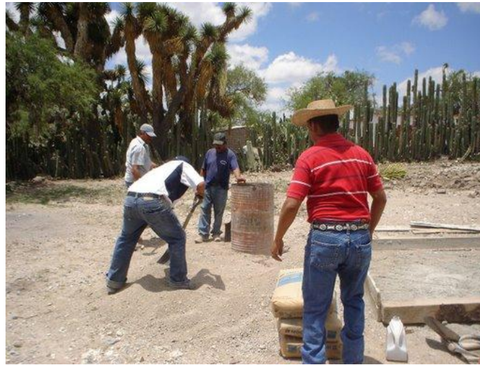
Platform being built by BYOW Water Committee and other community men
