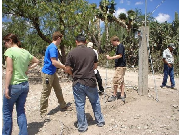
Electric wire grounded by the team from the BYOW location to the electric grid
